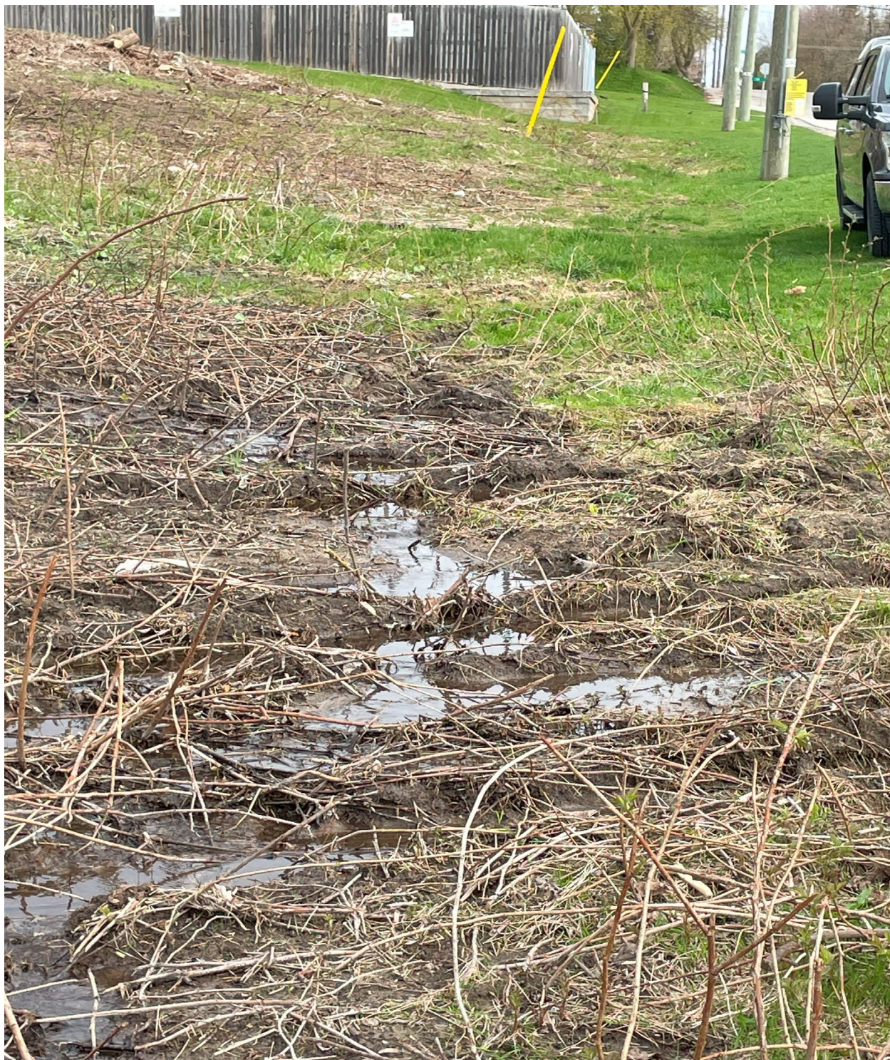
Surface water from seepage at toe of slope draining south May 5, 2025
